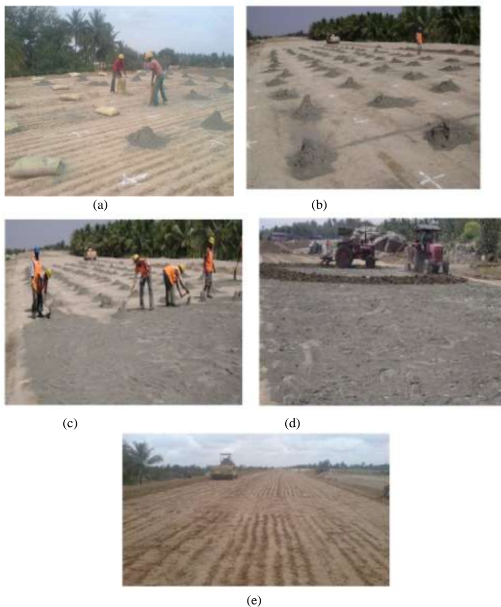
Figure 1: Showing cement stabilized subgrade at test site.
